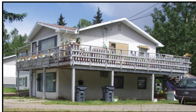
Photograph 4. This residence was located just outside of the Inverness trailer park and appears to be the typical way of storing automated garbage cans, even in this high bear destruction area (July 10, 2008).
