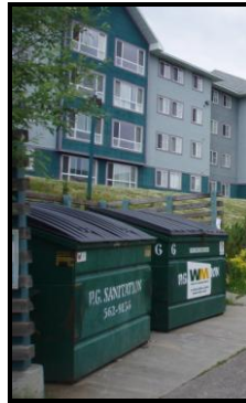
Photograph 25. This type of large bins pictured in the resident parking lot requires new lids to be bear-resistant.
